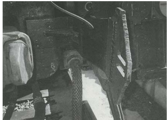
Photo 5: Under platform bracket (front view)
